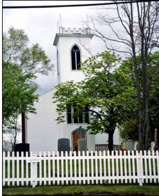
Figure 1: St. Stephen's Anglican Church, Chester, N.S.
