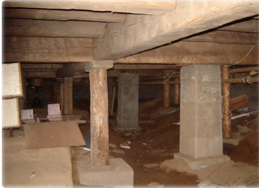
Figure 3. Basement of the St. Antoine-Padoue Church displaying axe-hewn beams.
